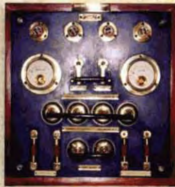
The Charging Panel used to charge the lead acid batteries.
