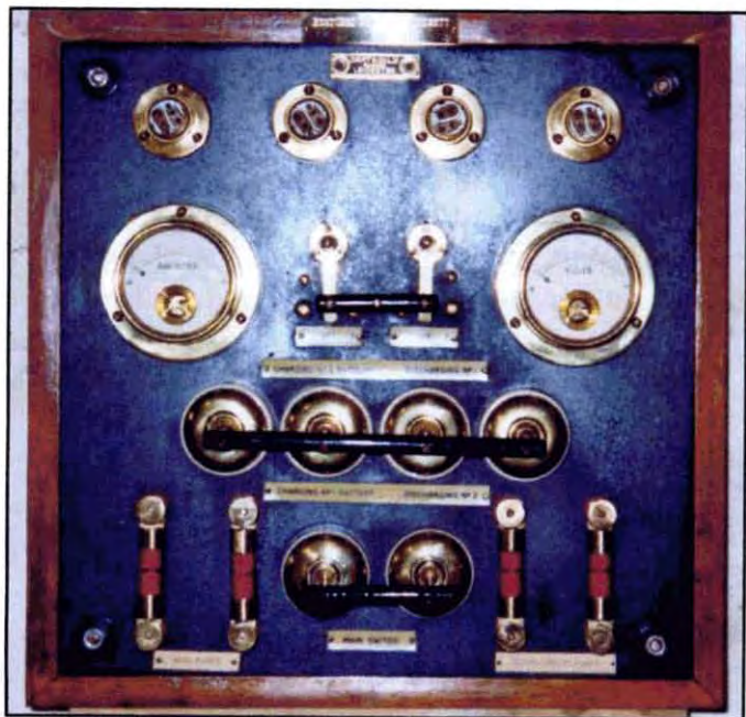
The restored Charging Panel.
